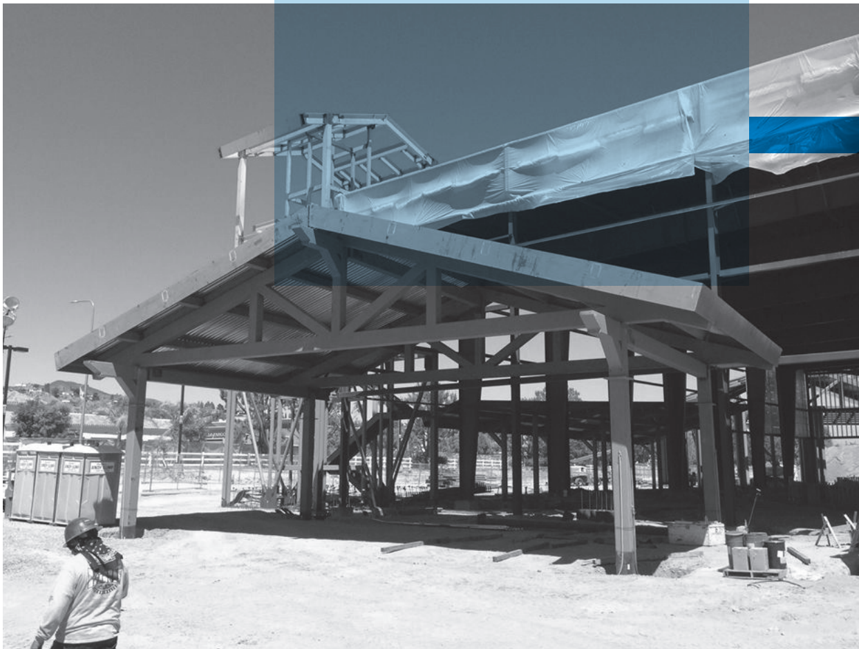
Construction Photos: Main steel truss column members (Gathering Pavilion/Bell-Tower)
