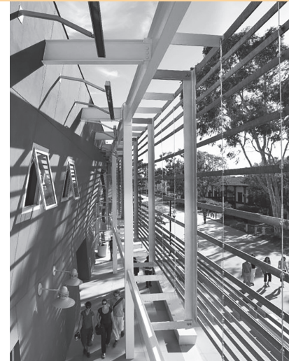
A-Built Facade Detail Photo
