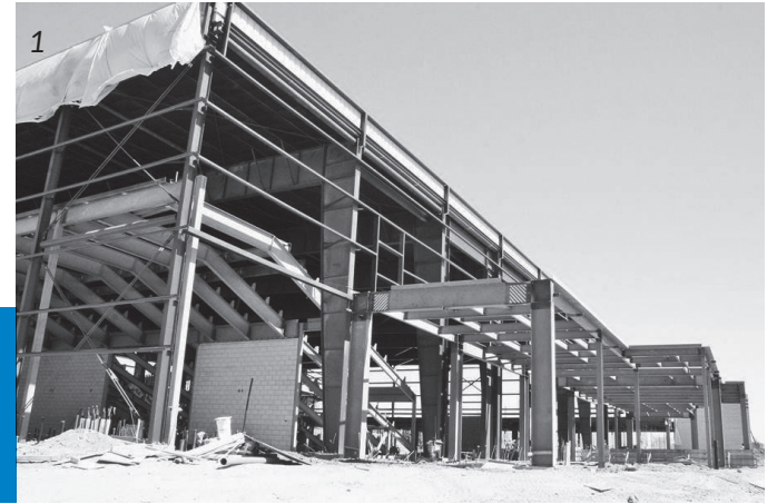
Construction Photos: Main steel truss column members (Gathering Pavilion/Bell-Tower)
